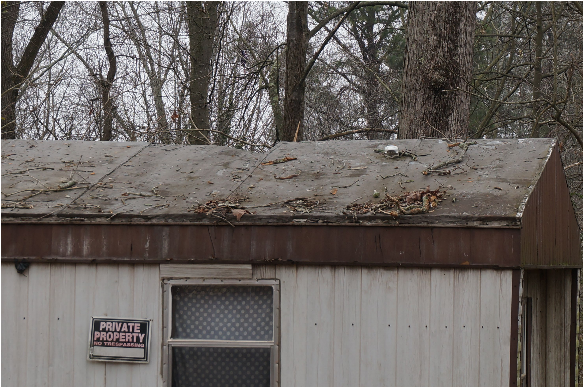
Photo 4 – Roof of Mobile Home
