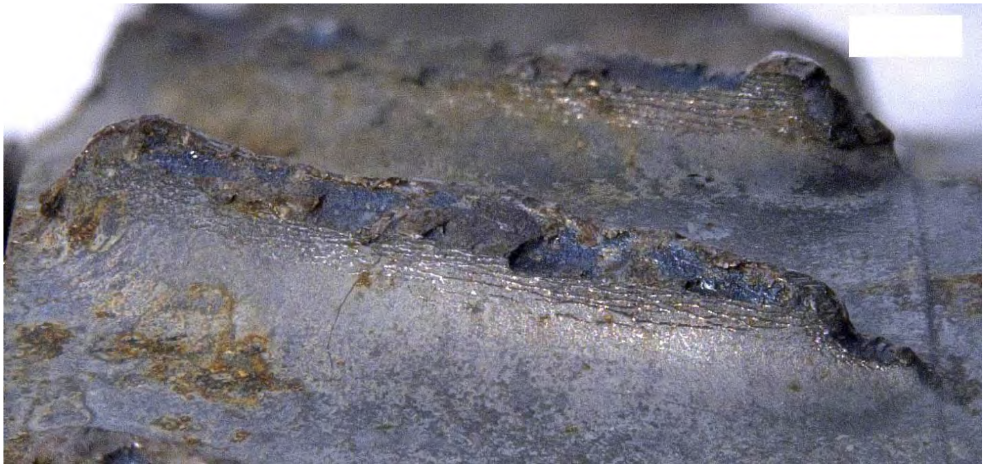
Figure 84. Detailed views of the fracture surface (top) and suction side surface (bottom) of stage 6 compressor blade 21 (see Figures 62 and 63). The red arrows indicate the local direction of fatigue progression. The yellow arrow indicates a ratchet mark consistent with fatigue initiation on the suction side surface.
