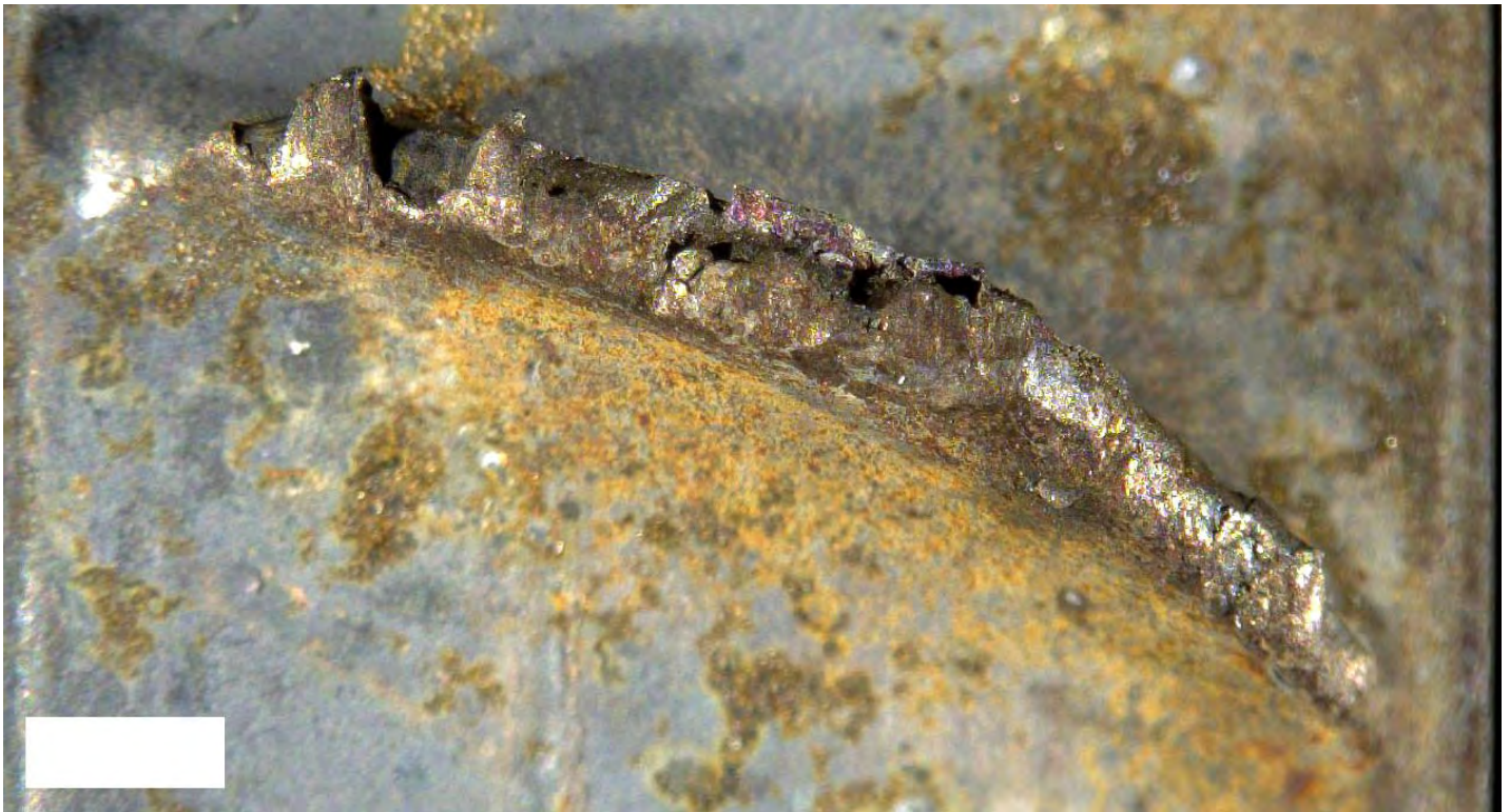
Figure 54. Detailed views of two stage 5 blade fracture surfaces. No fatigue fracture features were present on either of the fracture surfaces.
