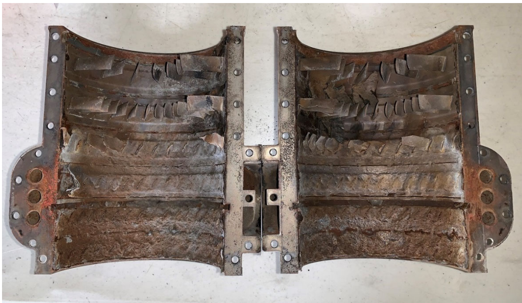
Figure 8. The two compressor case halves showing the damaged liner.
