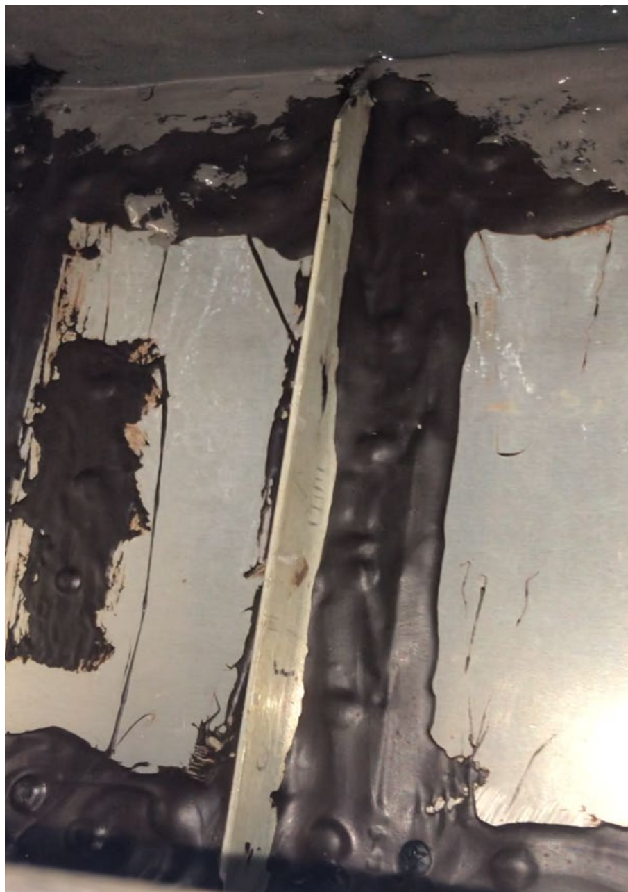
Photo 8 - Interior of Right Wing Fuel Tank – Courtesy of FAA
