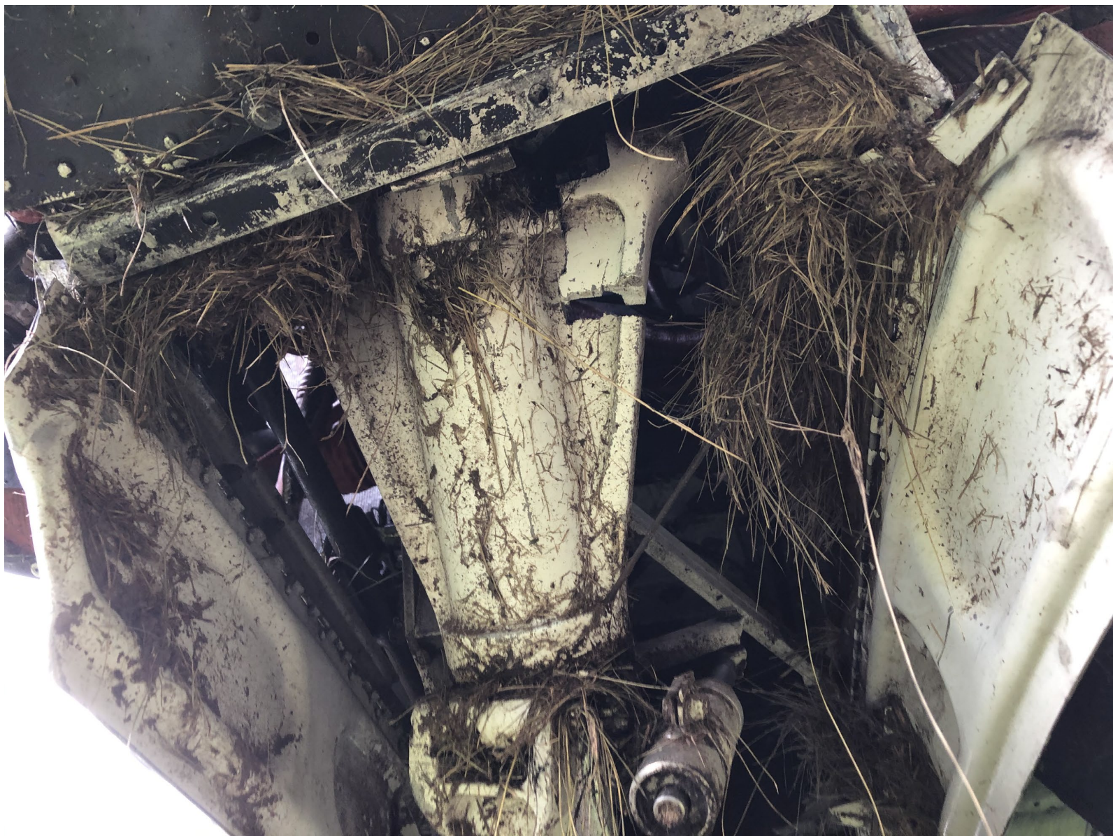
Photo 11 – Close Up of Displaced Nose Landing Gear – Courtesy of McLarens Adjusting
