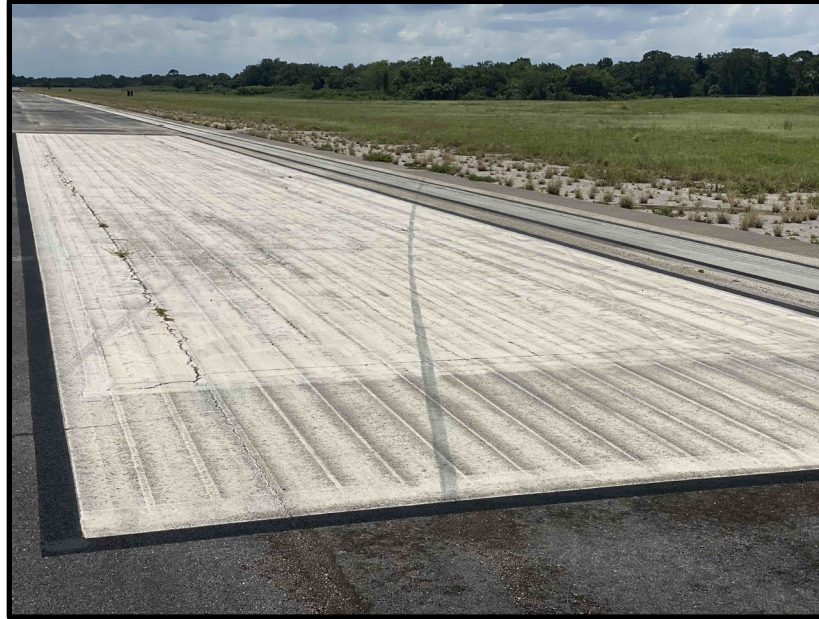
Figure 9-Rubber transfer marks on white Runway 27 right aiming point marking.
