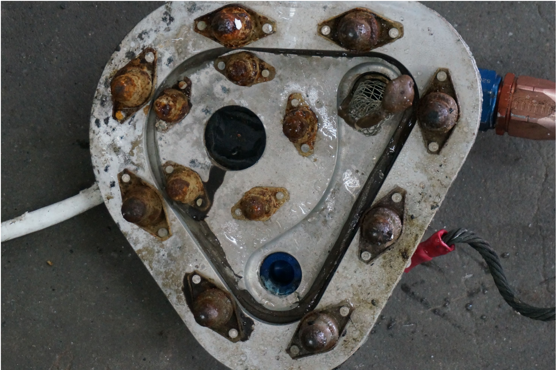
Photo 18 – Fuel Tank Sump Flange (Probe Side)
