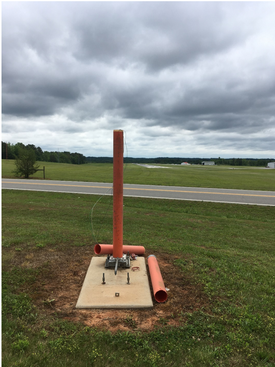
Figure: Digital Photograph Provided by Pilot Depicting Impacted Obstruction Light Pole in Foreground and Approach End of Runway in Background.
