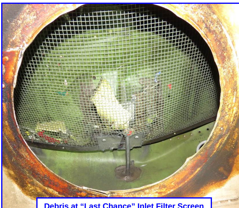
Debris at "Last Chance" Inlet Filter Screen
