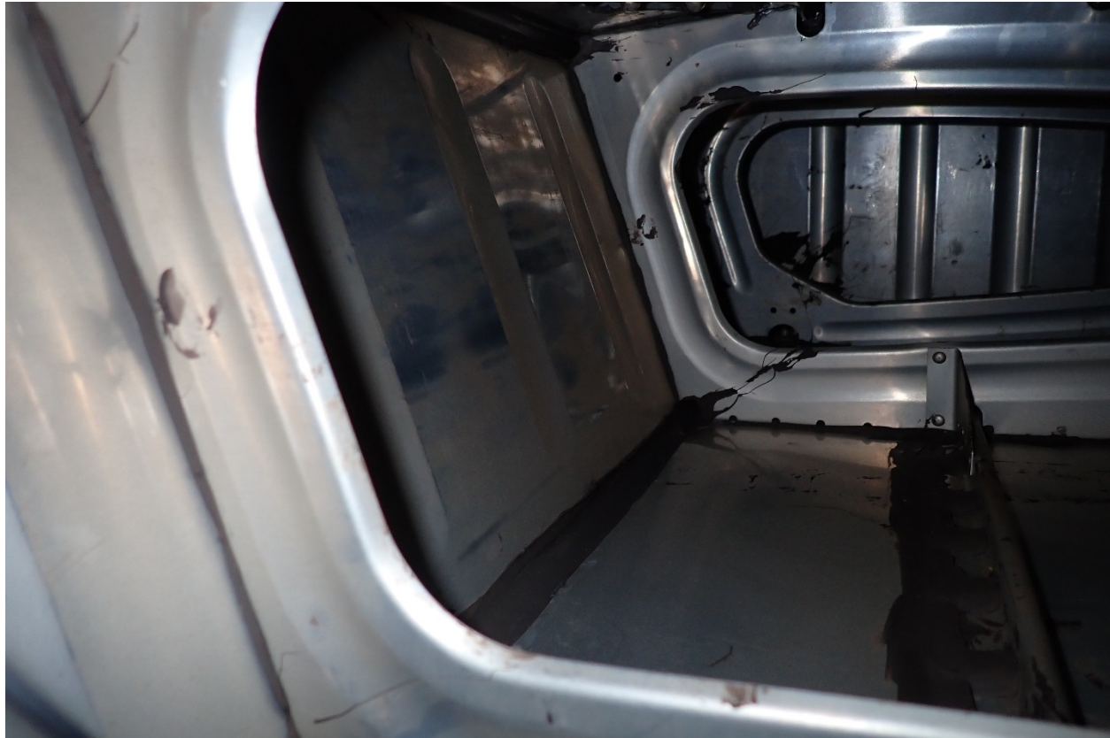
Figure 2 Inside of Right Wing Fuel Tank - Lowest Corner
