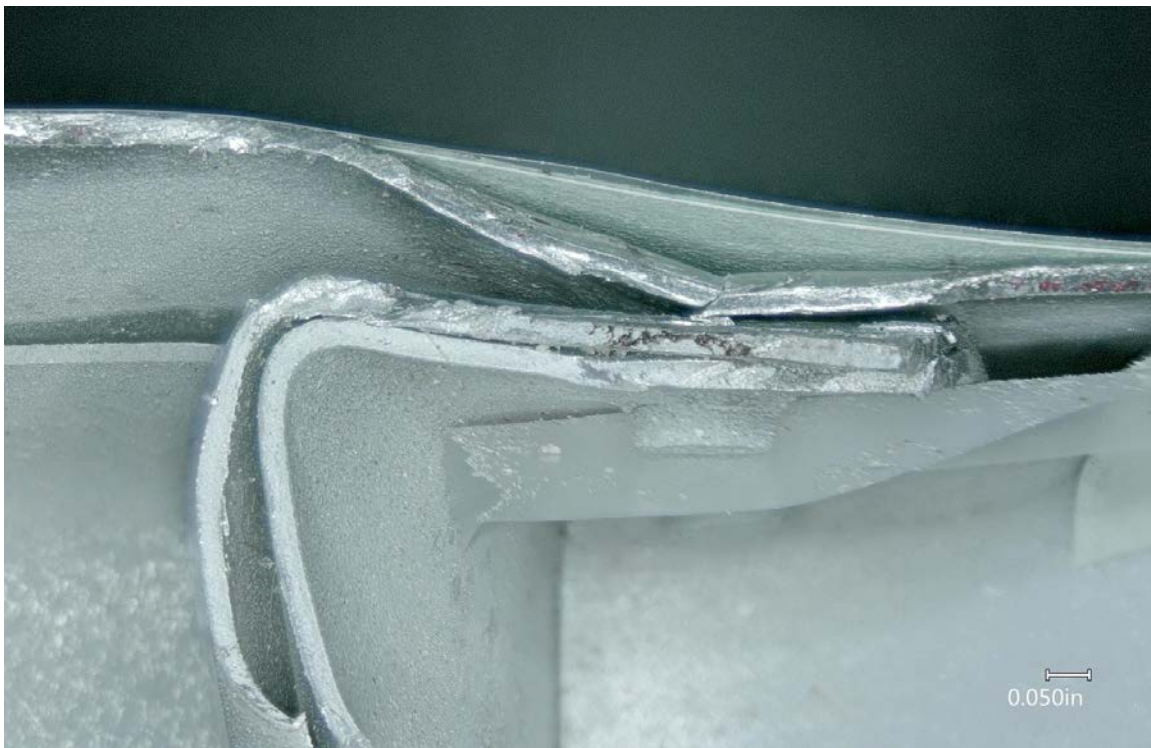
Figure 7: A close-up photo (top) and digital microscope image (bottom) of a flat area on the fracture surface at the corner of the doubler.
