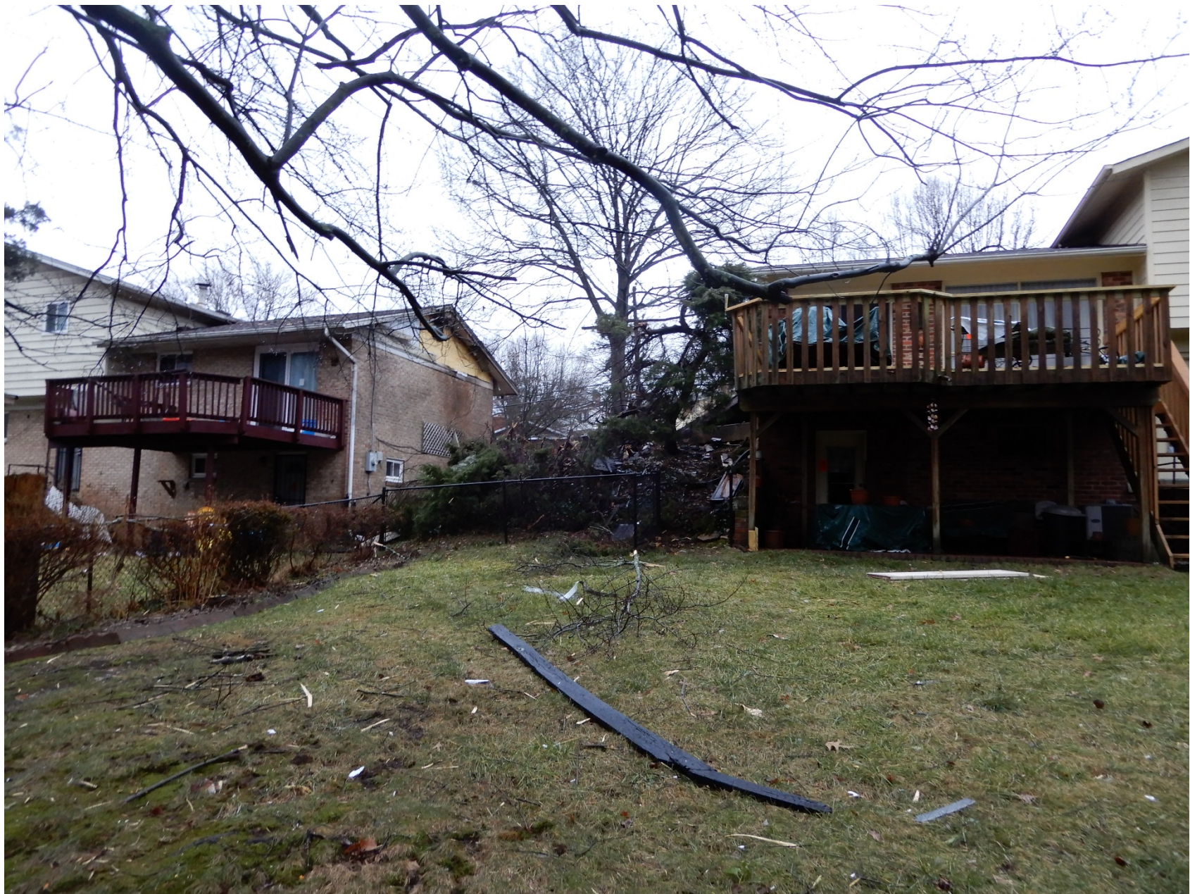
Photo 1 – View of the initial impact point, between two houses.
