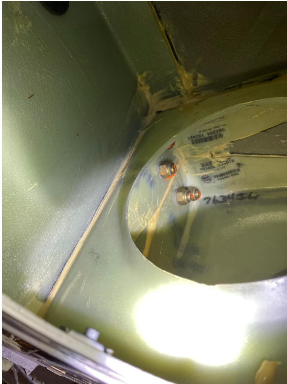
Photo 3 – Delamination of Wing Spar (Photo Courtesy of FAA)
