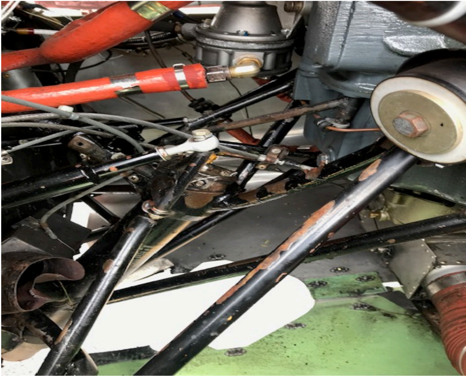
Photo 3 - Courtesy of FAA- showing buckled engine mount
