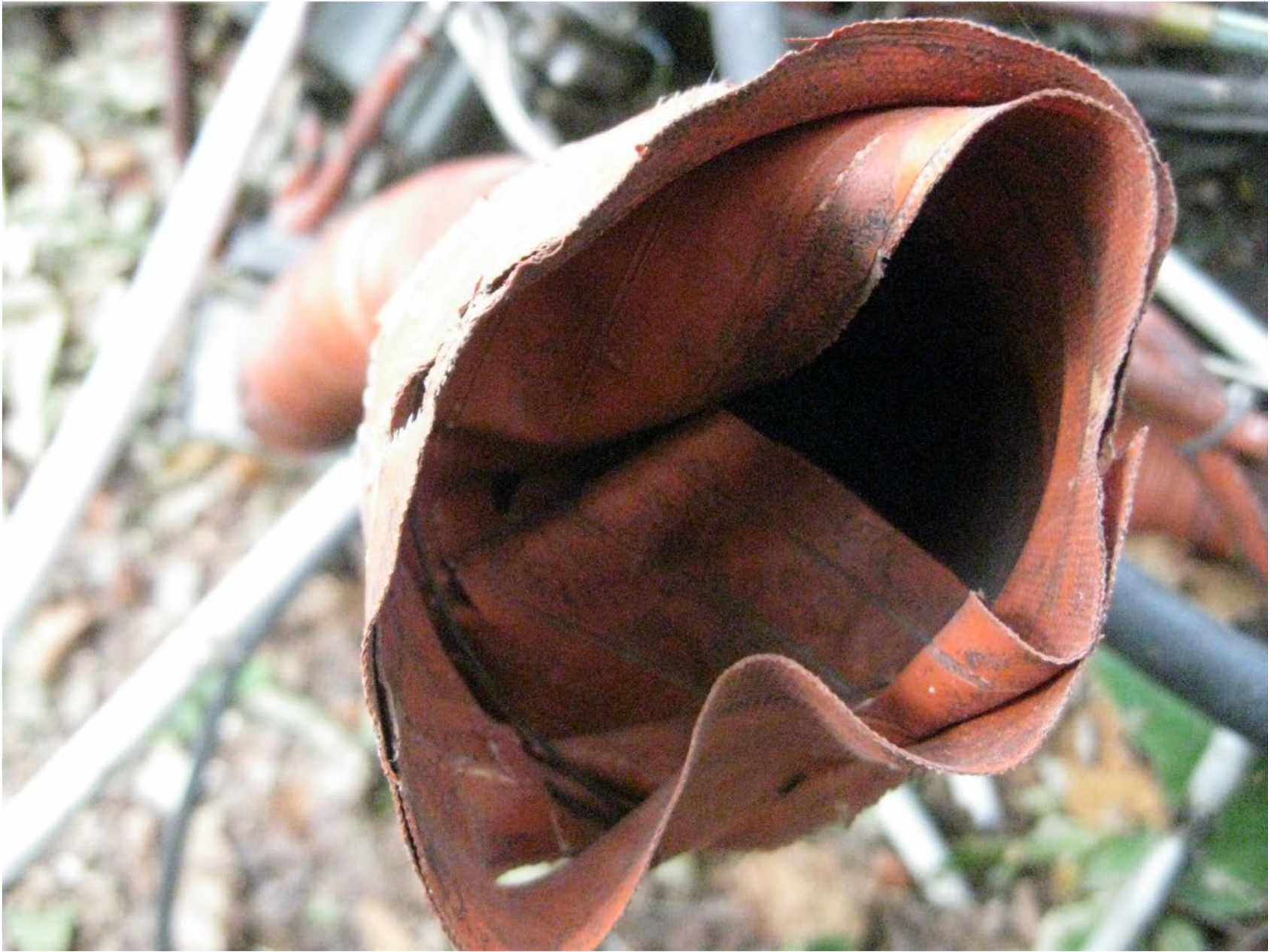
Photo 2 – View of inside of scat tubing showing the collapsed inner layer
