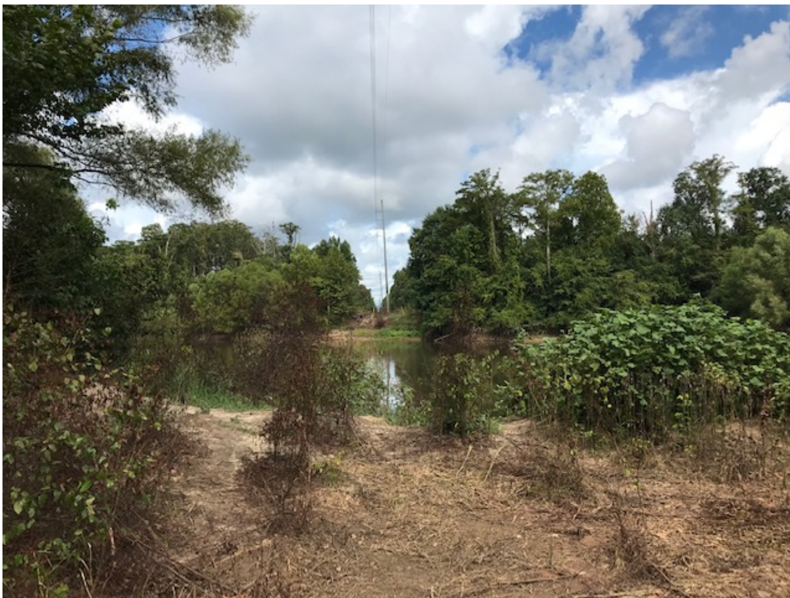
Photo 7 – Photograph of transmission lines over the water looking west from the bank of the river. (Courtesy of Maverick Natural Resources, LLC)
