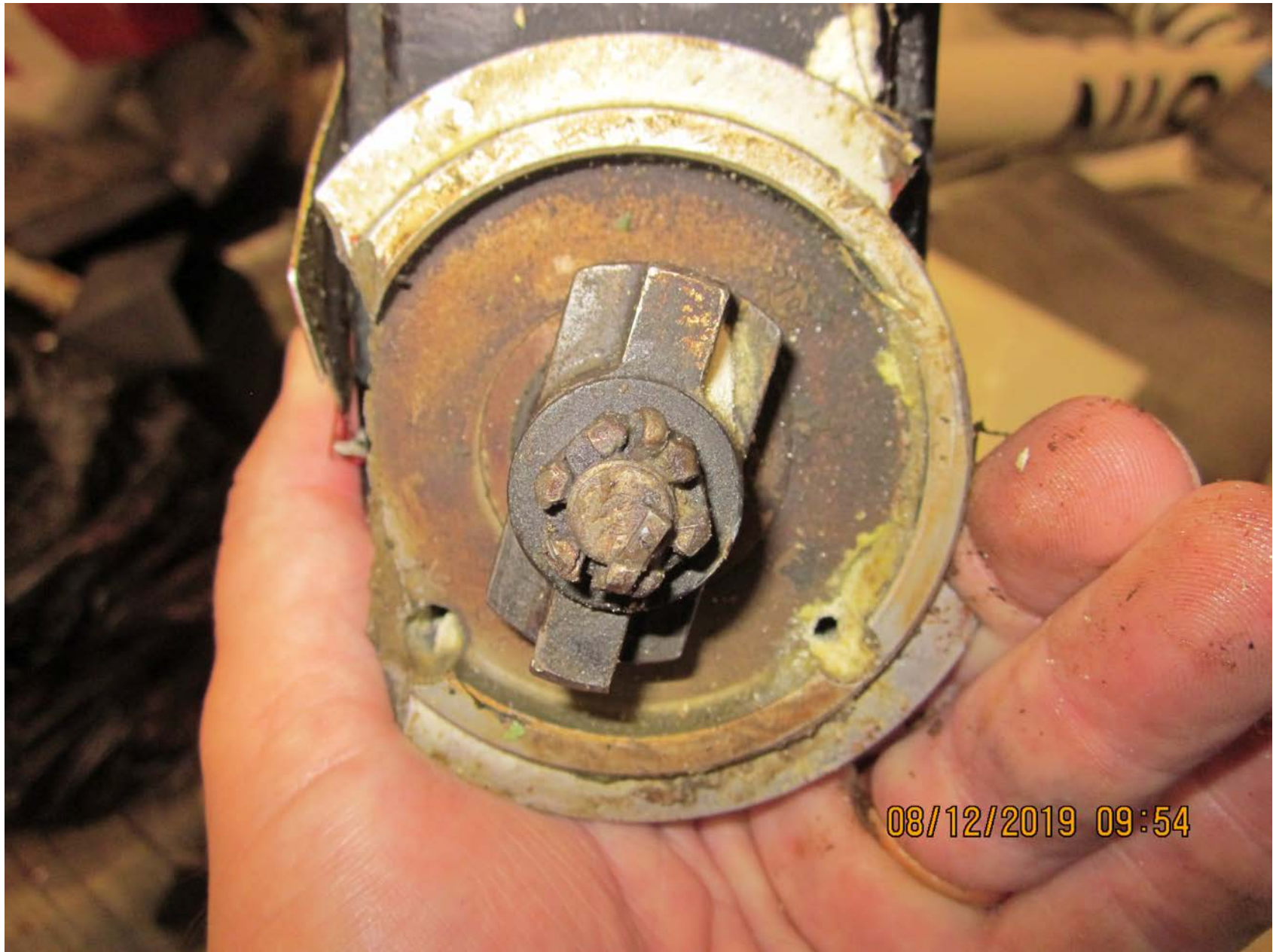
Photo 4 – View of corrosion within the right magneto
