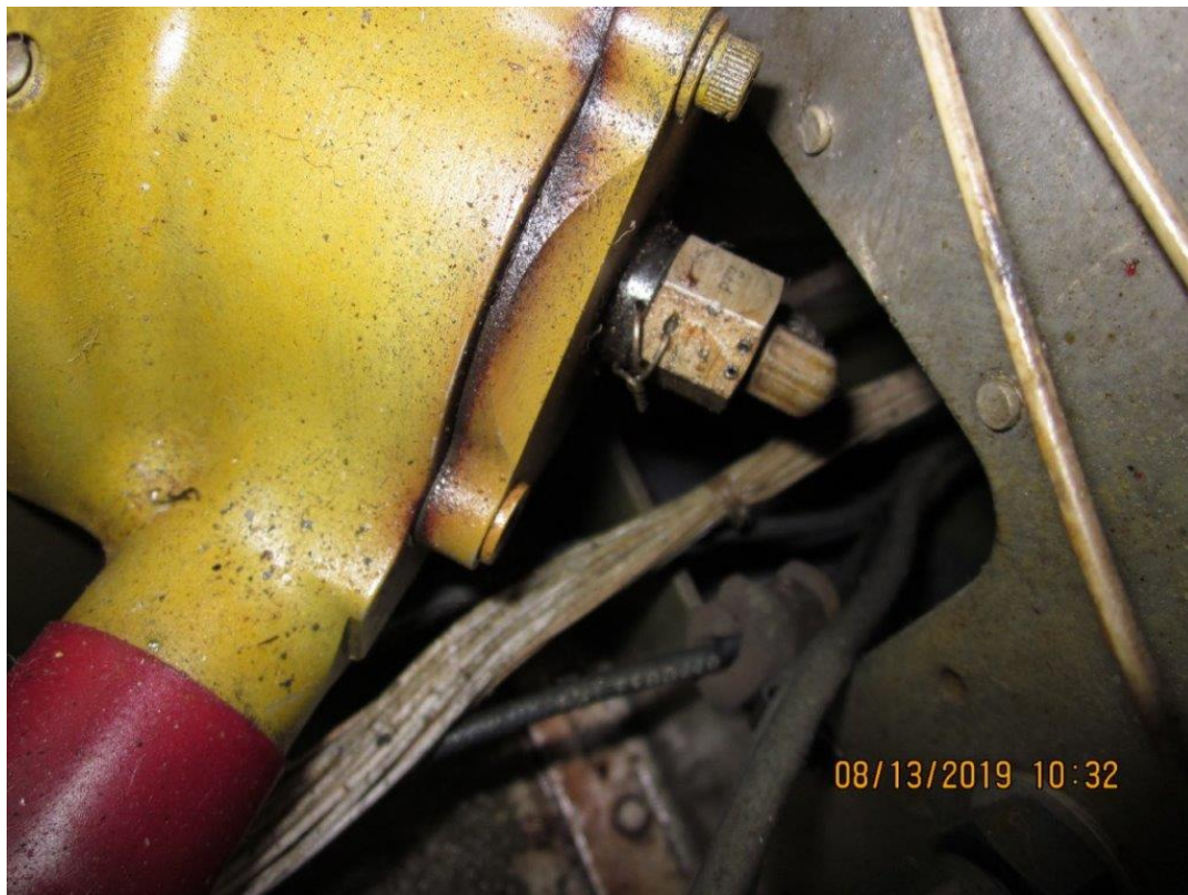
Figure 1: Sheared Screw Head from the Actuator End Cap (Photo Courtesy of FAA)
