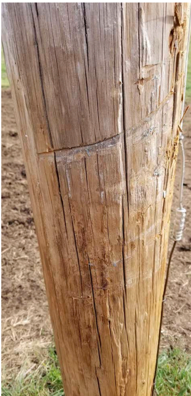
Photo 2 – FAA Digital Photograph. View of the Power Pole Contacted By the Left Wing.
