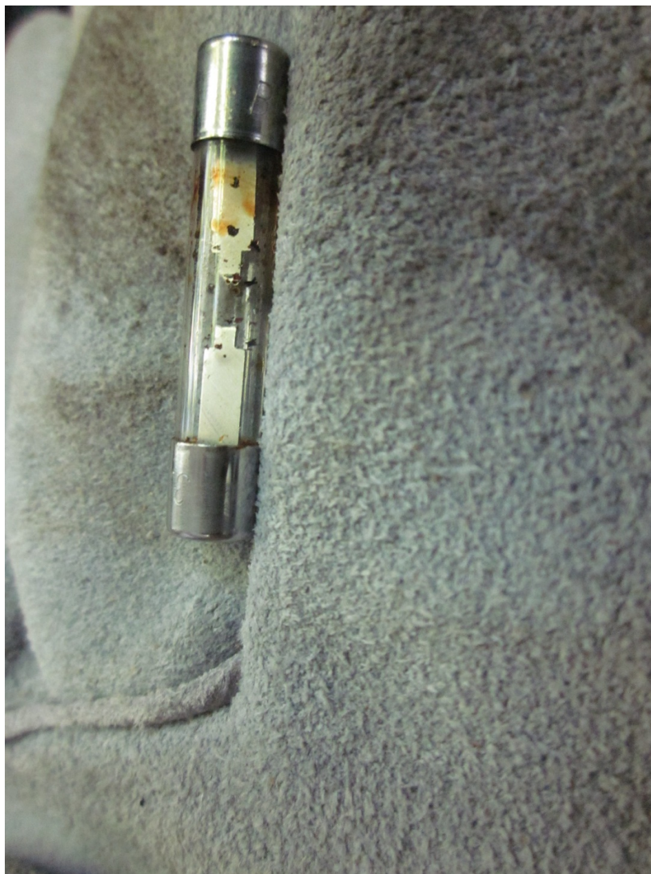
Photo 3 – Spare Fuse Blown as Found by FAA Inspector (Photo Courtesy of FAA)
