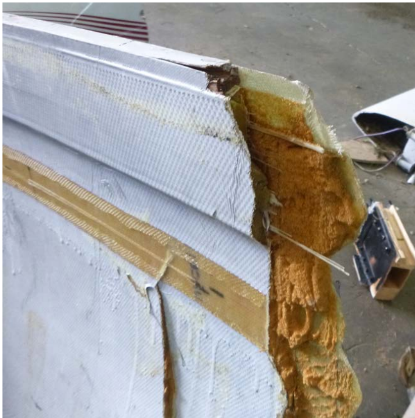
Figure 4 – Right longeron fracture, forward fuselage section
