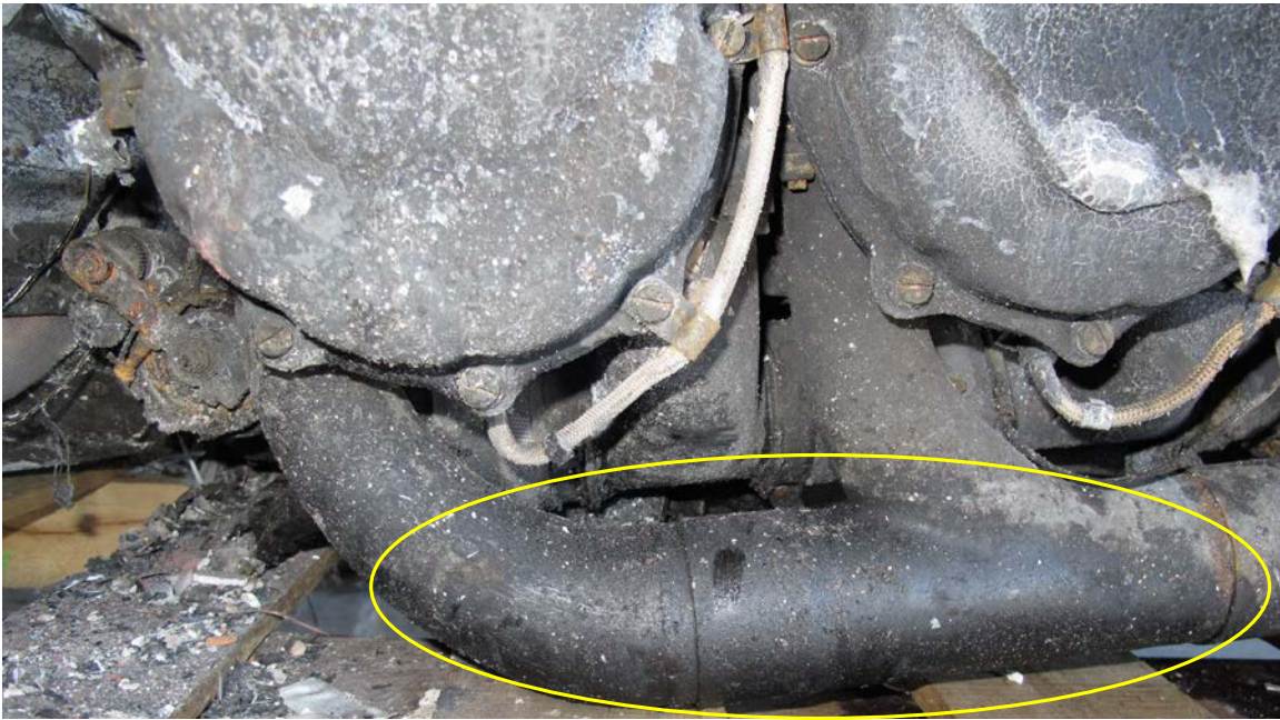
Figure 3. Close-up of oil staining (highlighted by yellow circle) left engine exhaust duct (#2, #4 and #6 cylinders' side).
