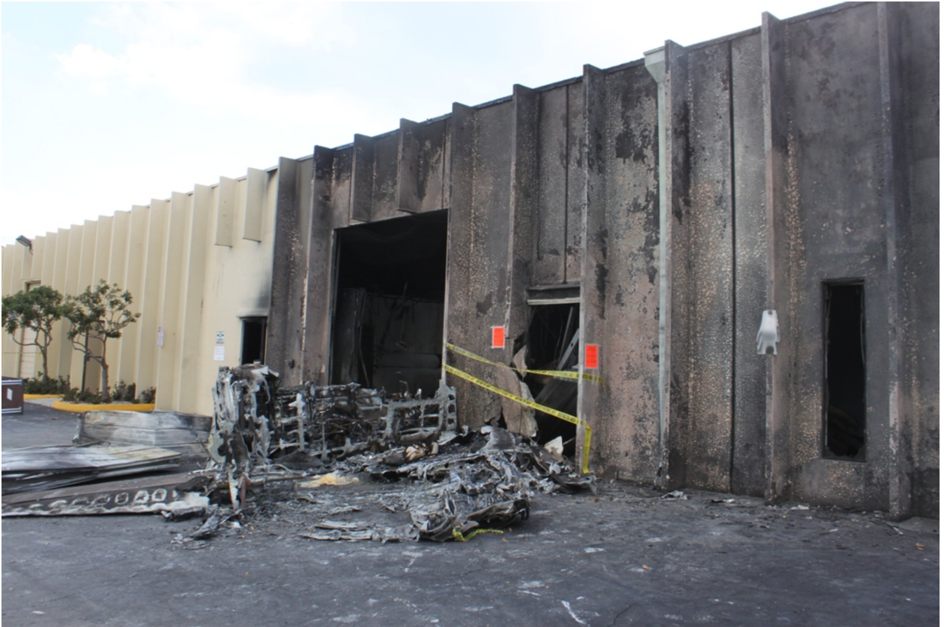
Photo 2 - NTSB Digital Photograph. Right Rear Quartering View Depicting Wreckage in Relation to Impacted Building.
