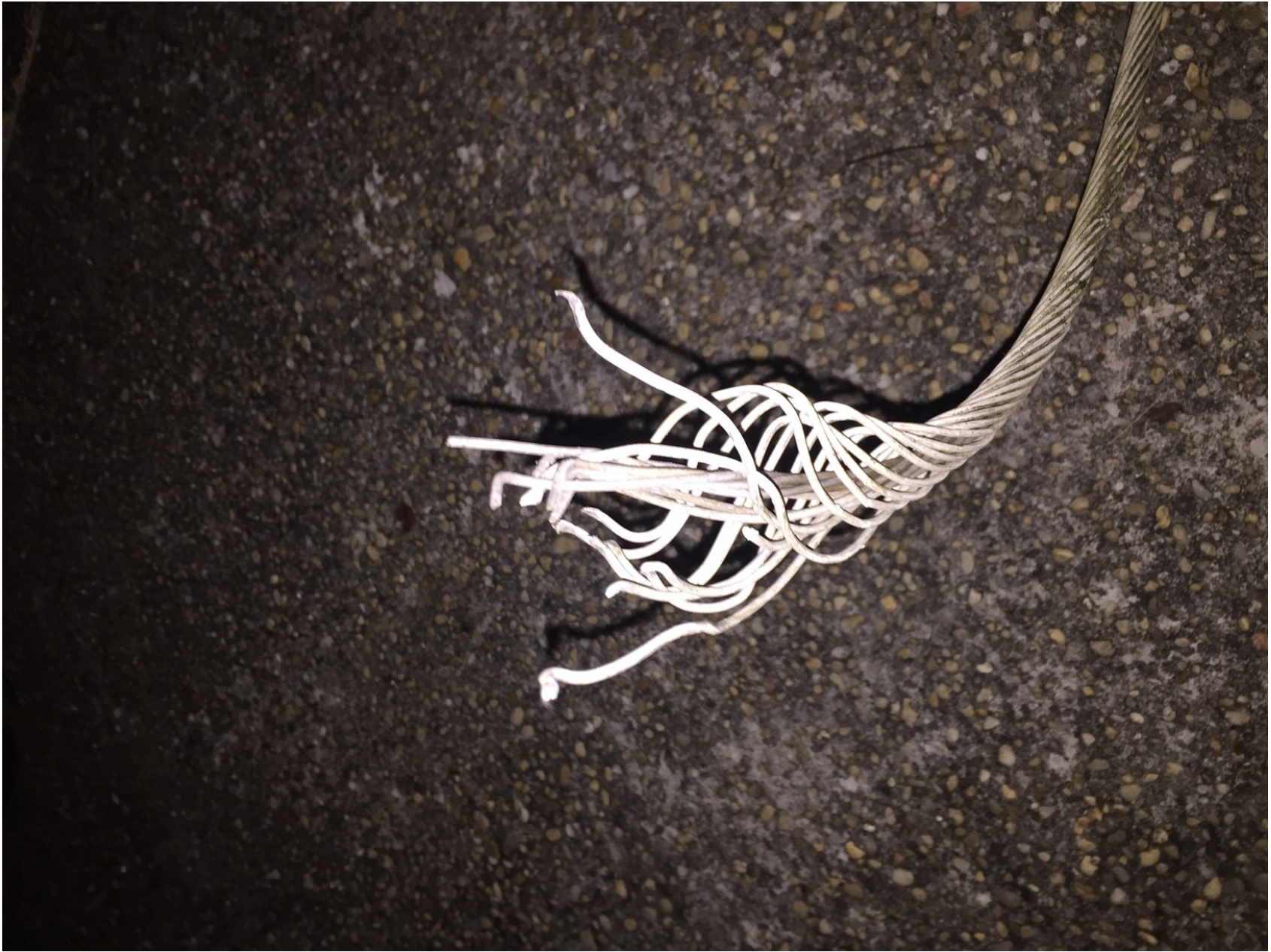
Photo 1 – View of the severed power lines.
