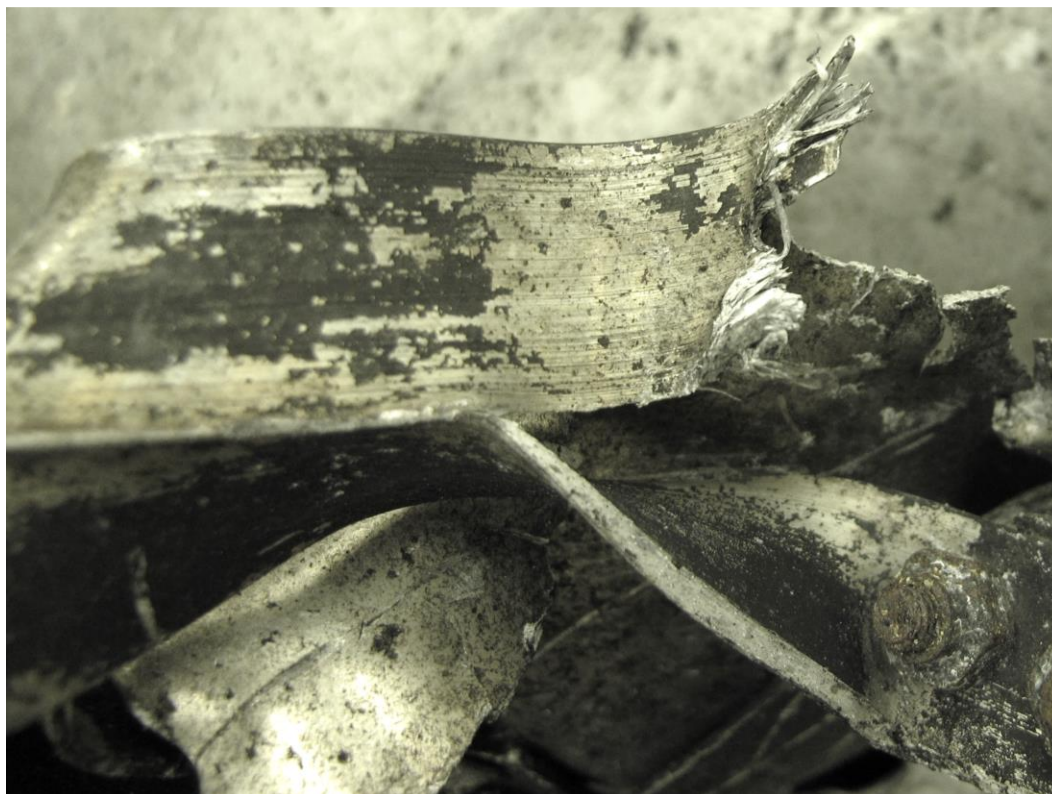
Figure 4. Close-up photograph of second area of broomstrawing.
