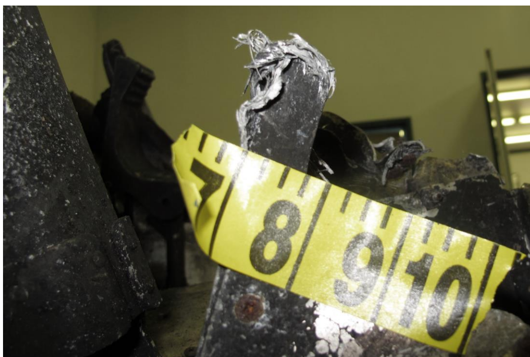
Figure 2. Area of broomstrawing on pedestal structure (side view).
