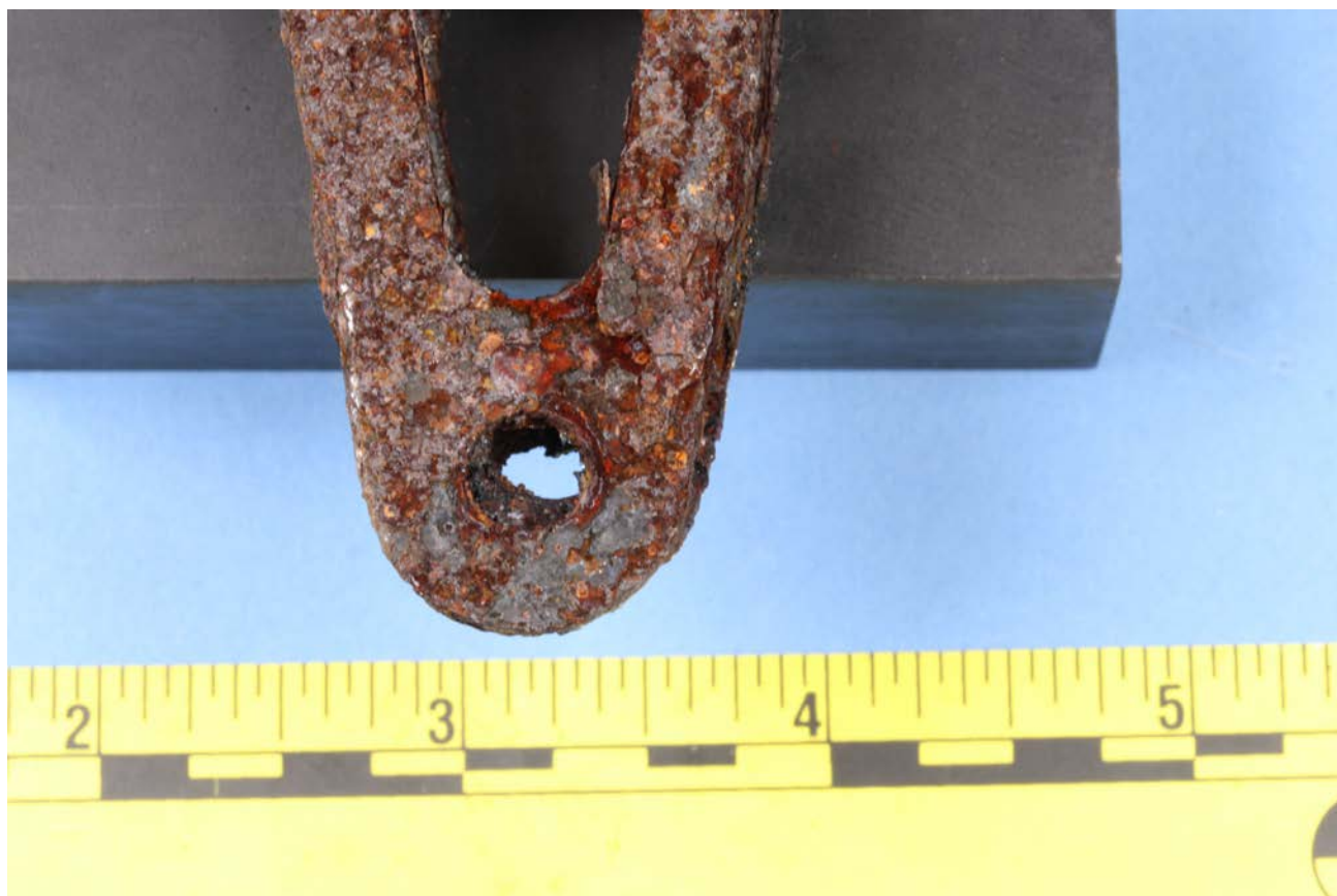
Figure 3: Clevis pin hole corroded but not deformed.
