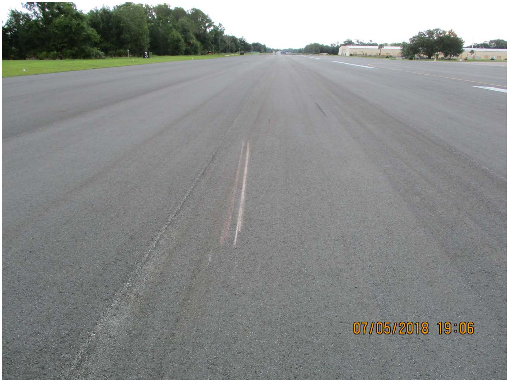
Photo 6 - Runway marks from left main landing gear.
