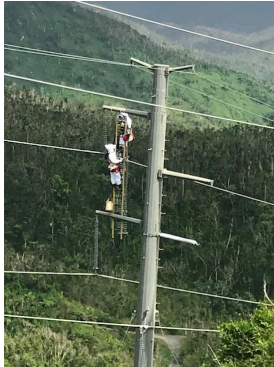
Lineman 1 & Lineman 2 on Pole 2 11 January 2018
