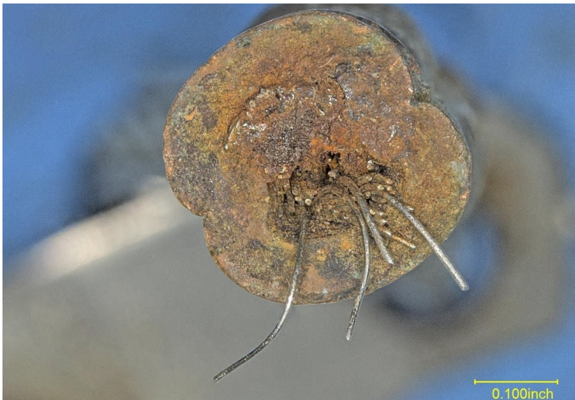
Figure 2 – View of the fractured cable bundle from the crimped fitting, highlighted in Figure 1.
