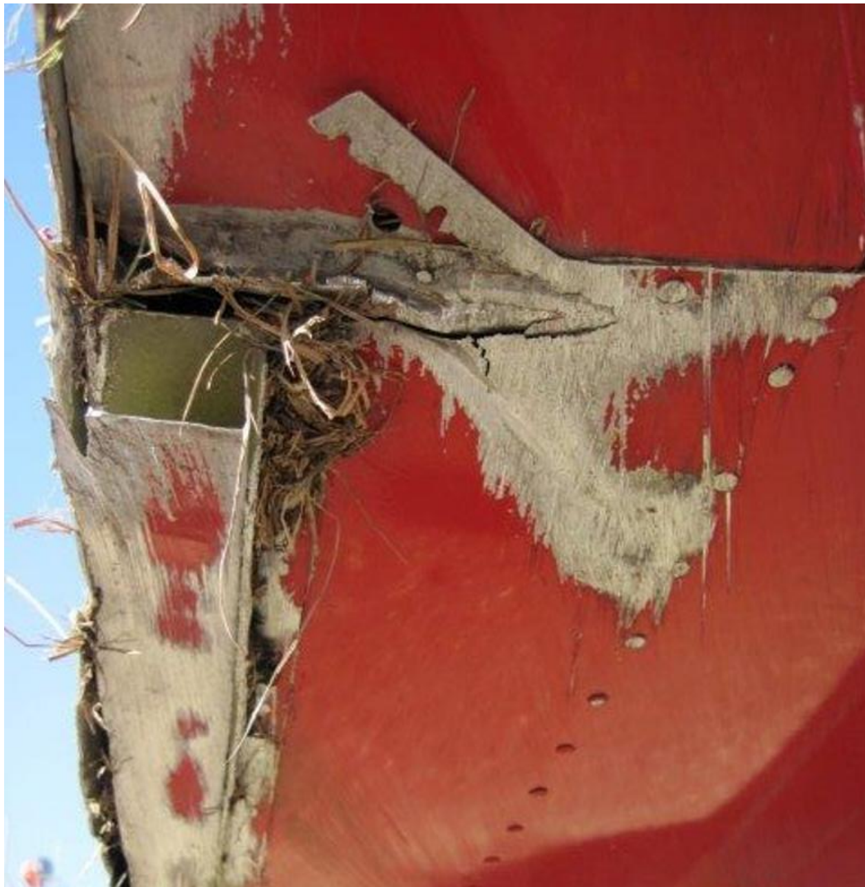
Photo 3 – Airframe Structural Damage (FAA Photo)
