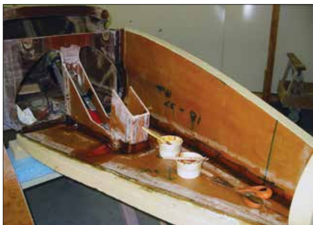
The inside of most of the nose is a box structure; this is the beginning of the nose.
