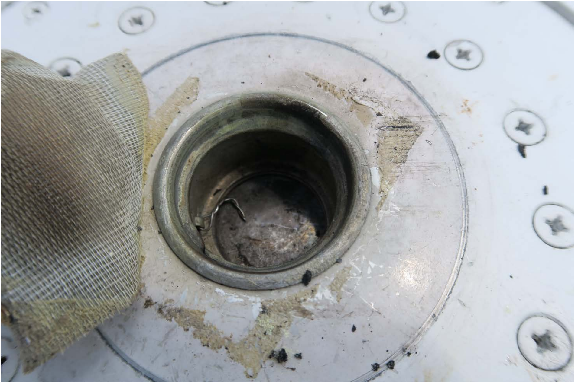
Photo 10 – View of right fuel port filler with tape peeled back for inspection, showing broken safety wire
