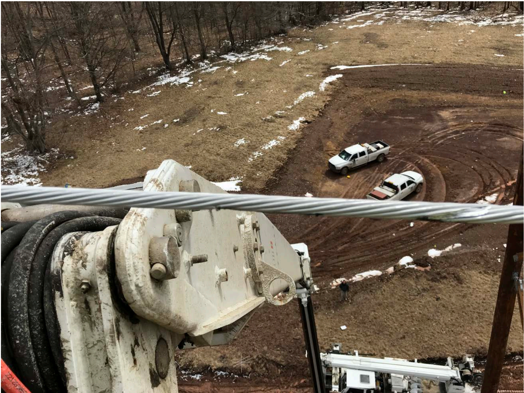
Photo 5 – View of Blemish on Static Line (Didado)
