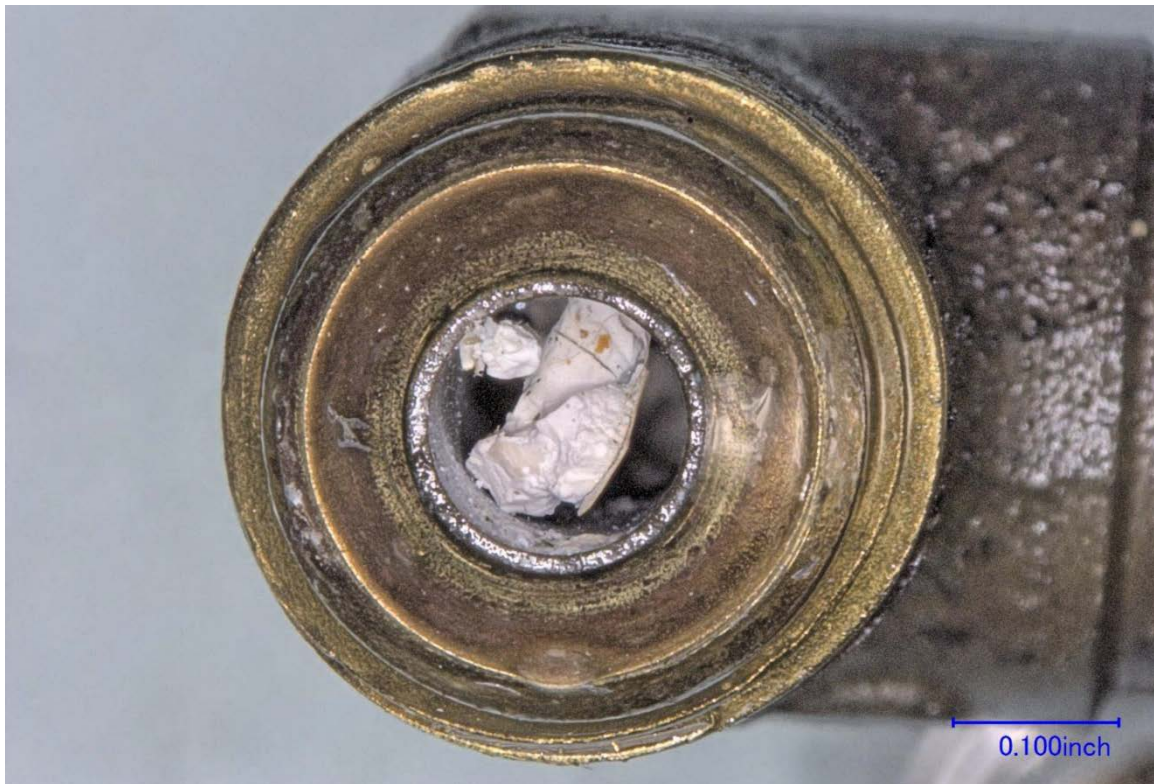
Figure 3 – Closer view of the 1.5 fitting orifice, showing white-colored material inside.
