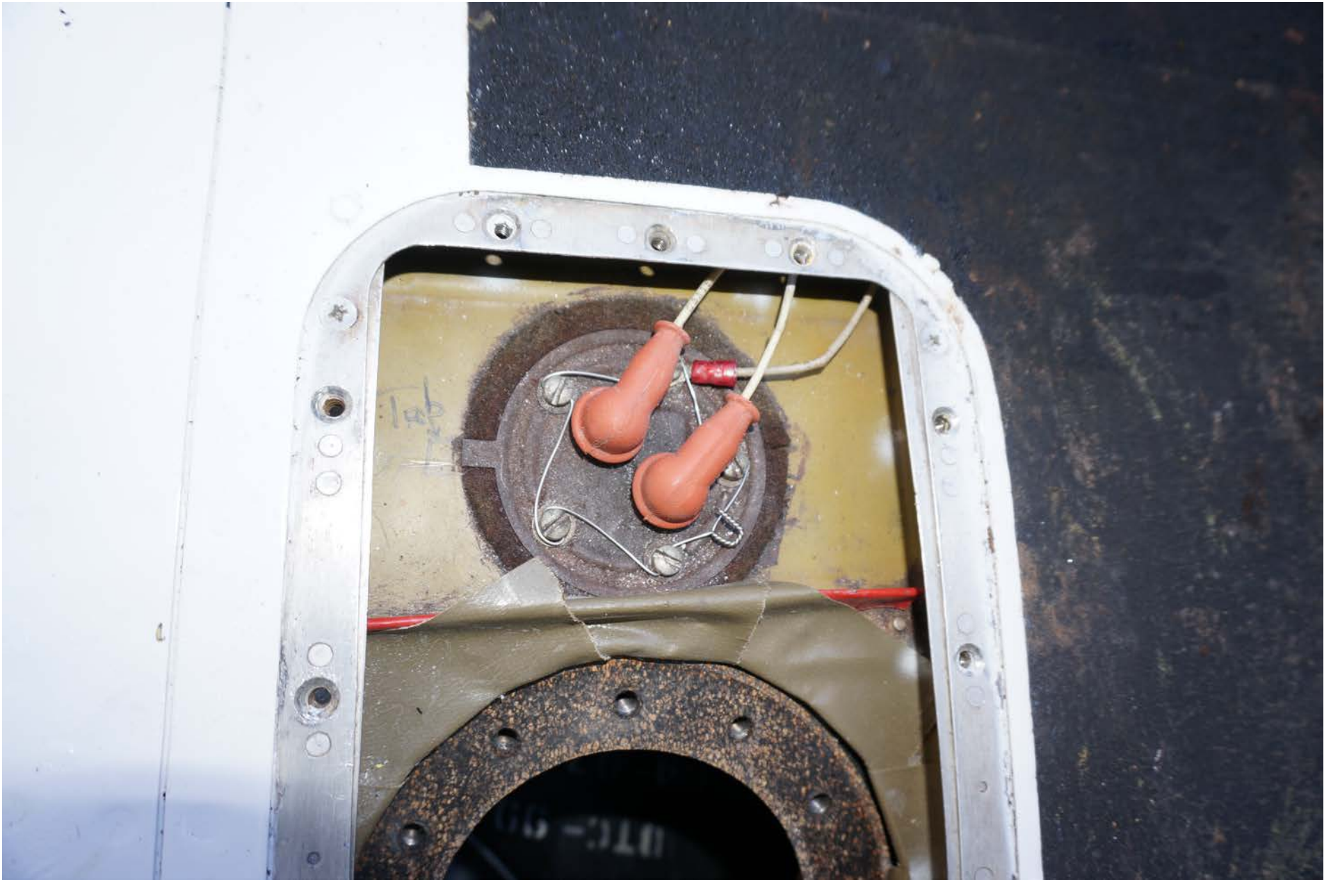
Photo 13 – Top of Right Fuel Tank Inboard Transmitter
