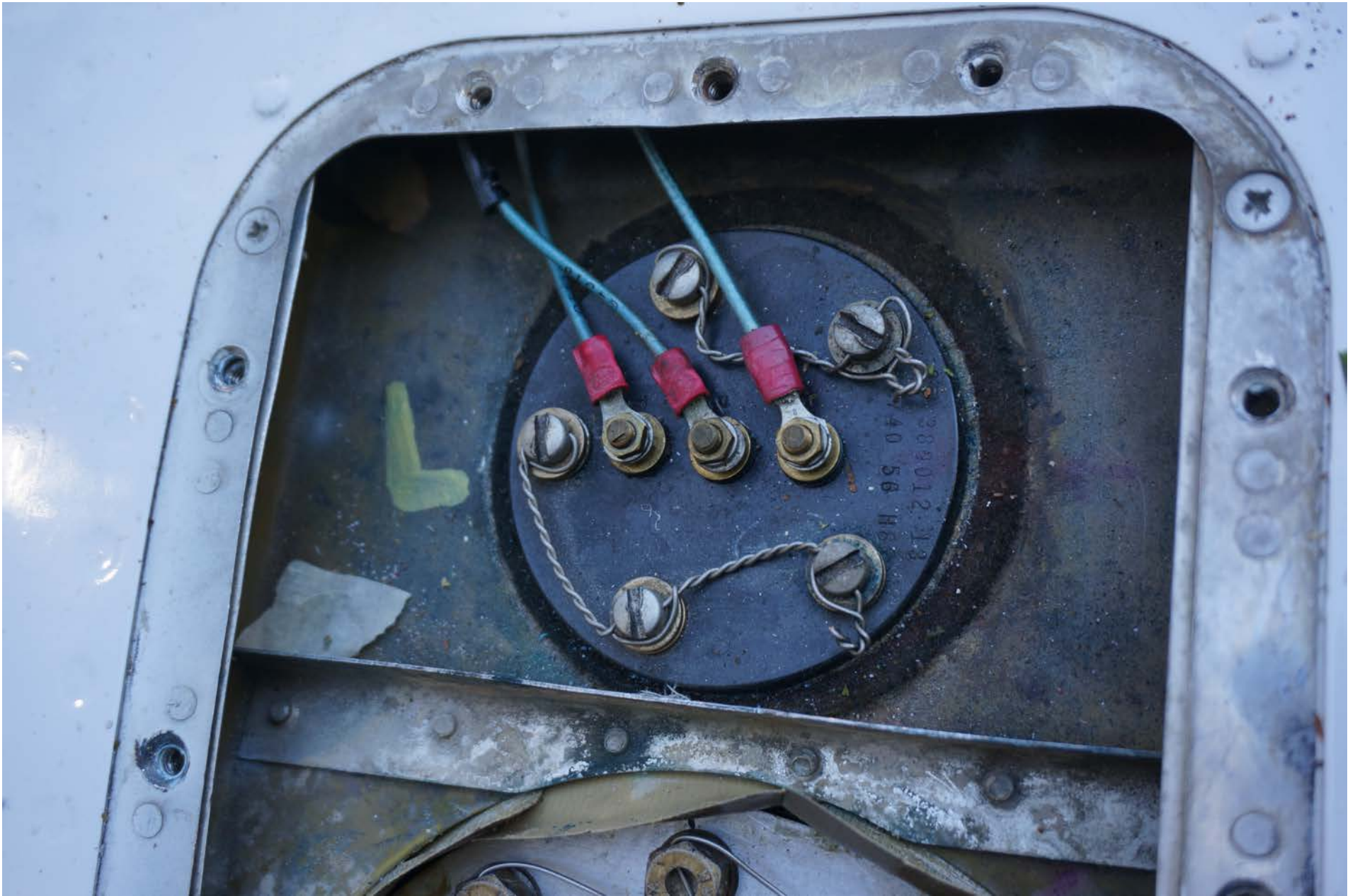
Photo 14 – Top of Left Fuel Tank Inboard Transmitter
