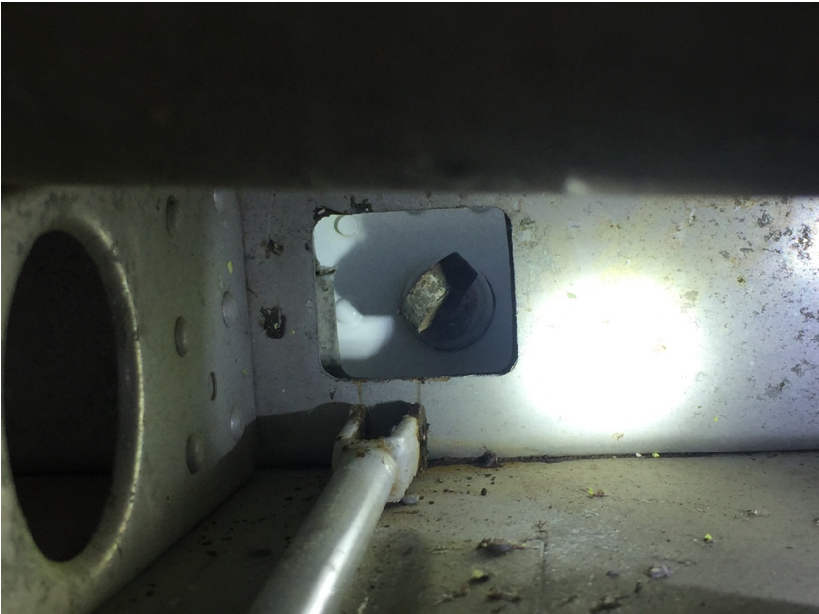
Photo 10 - Digital Photograph From FAA. View Inside the Right Elevator Depicting the Elevator Trim Push Rod Assembly Separated from the Trim Tab Actuator. Note the Rod Aft Of the Actuator and Main Spar of the Elevator.
