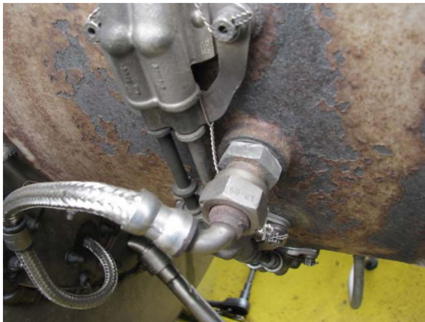
Photo No. 46 The other ignitor lead at the gas generator case
