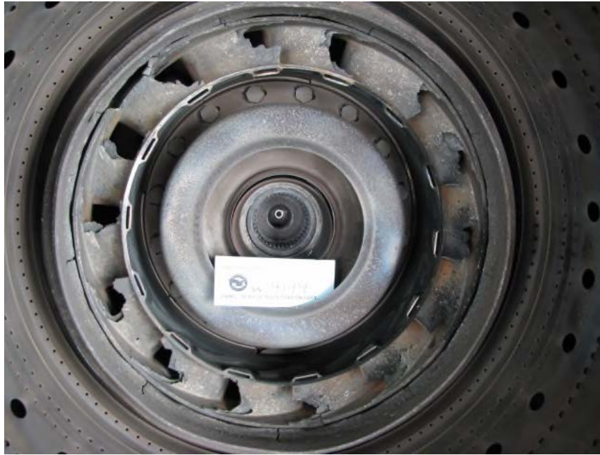
Photo No. 21 Compressor turbine stator downstream view
