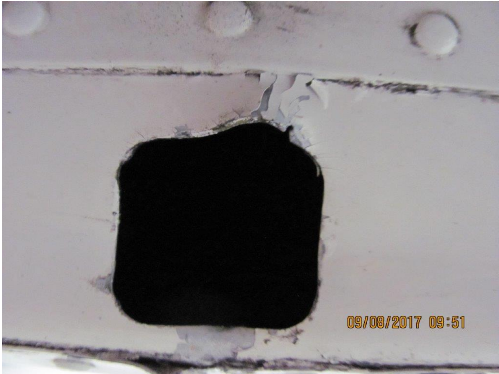
Photo 3 – View of Deformed/Fractured Aileron Control Rod Pass-Thru Hole (State of Vermont)
