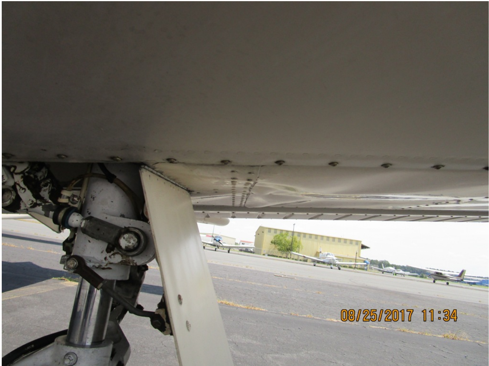
Photo 4 – Lower Left Wing Damage (Photo Courtesy of FAA)
