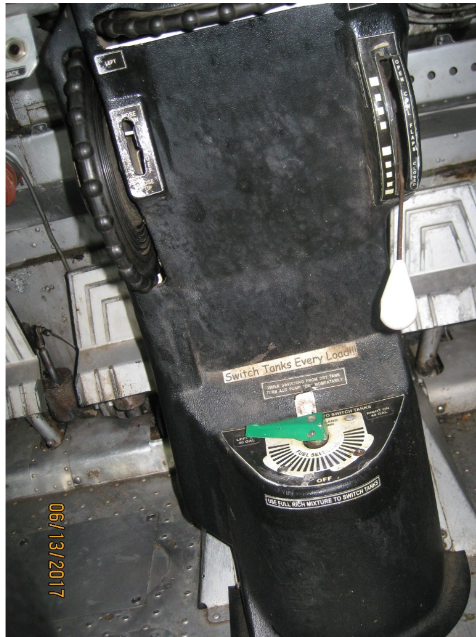
Photo 4 - FAA Digital Photograph. View of the As-Found Position of the Fuel Selector Valve.
