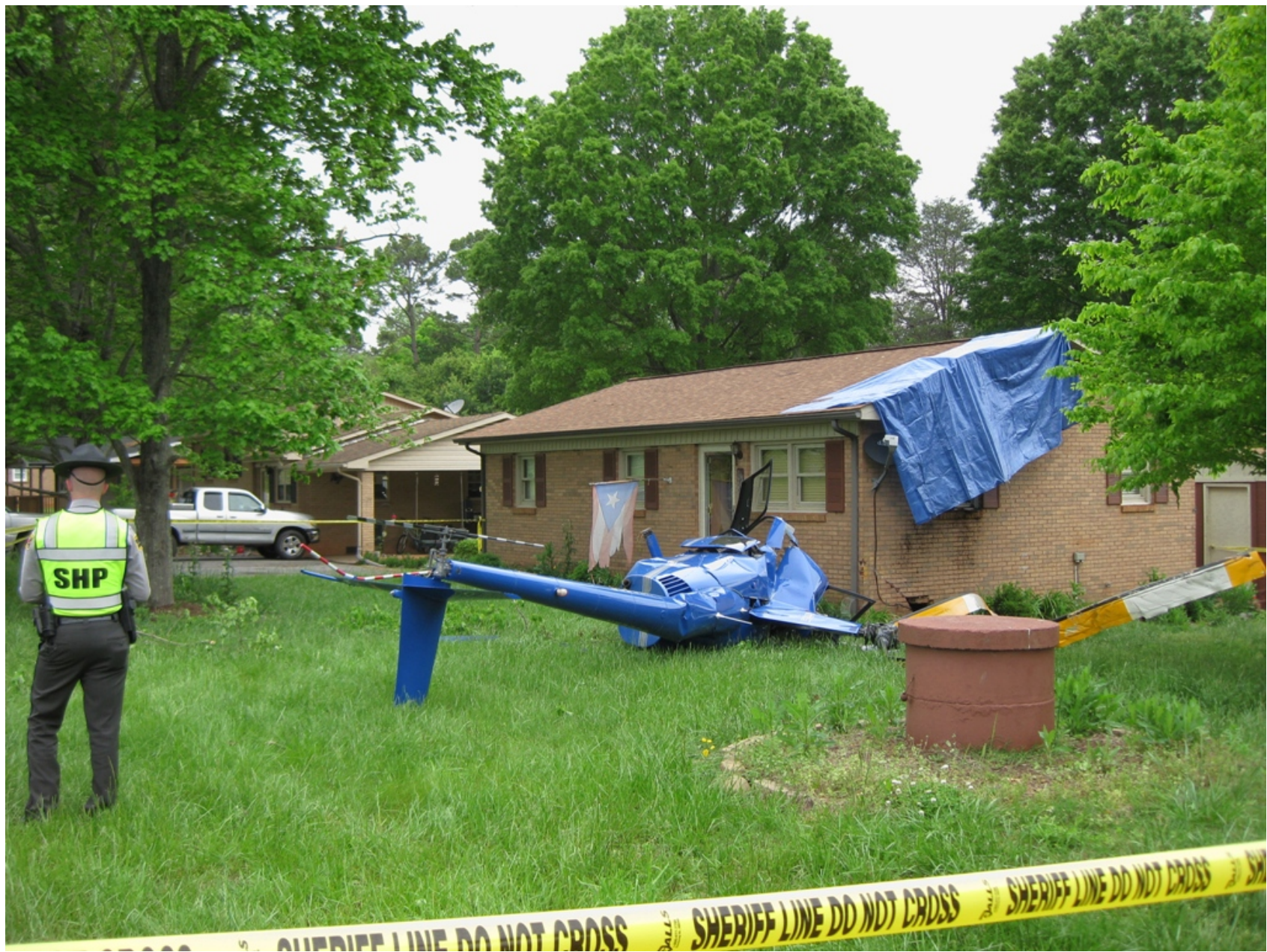
Photo 1 – Main Wreckage (Photo Courtesy of FAA)
