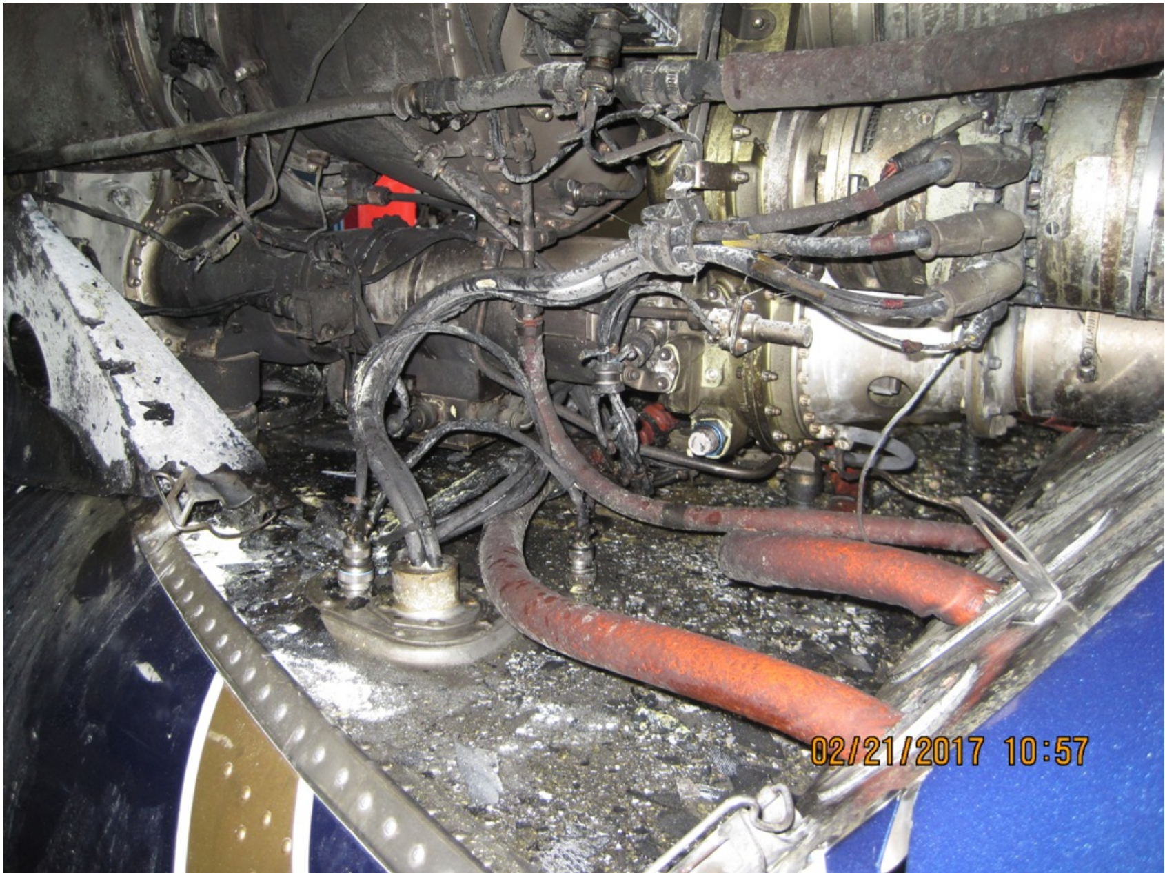
Photo 2 – Engine Deck (Photo Courtesy of FAA)
