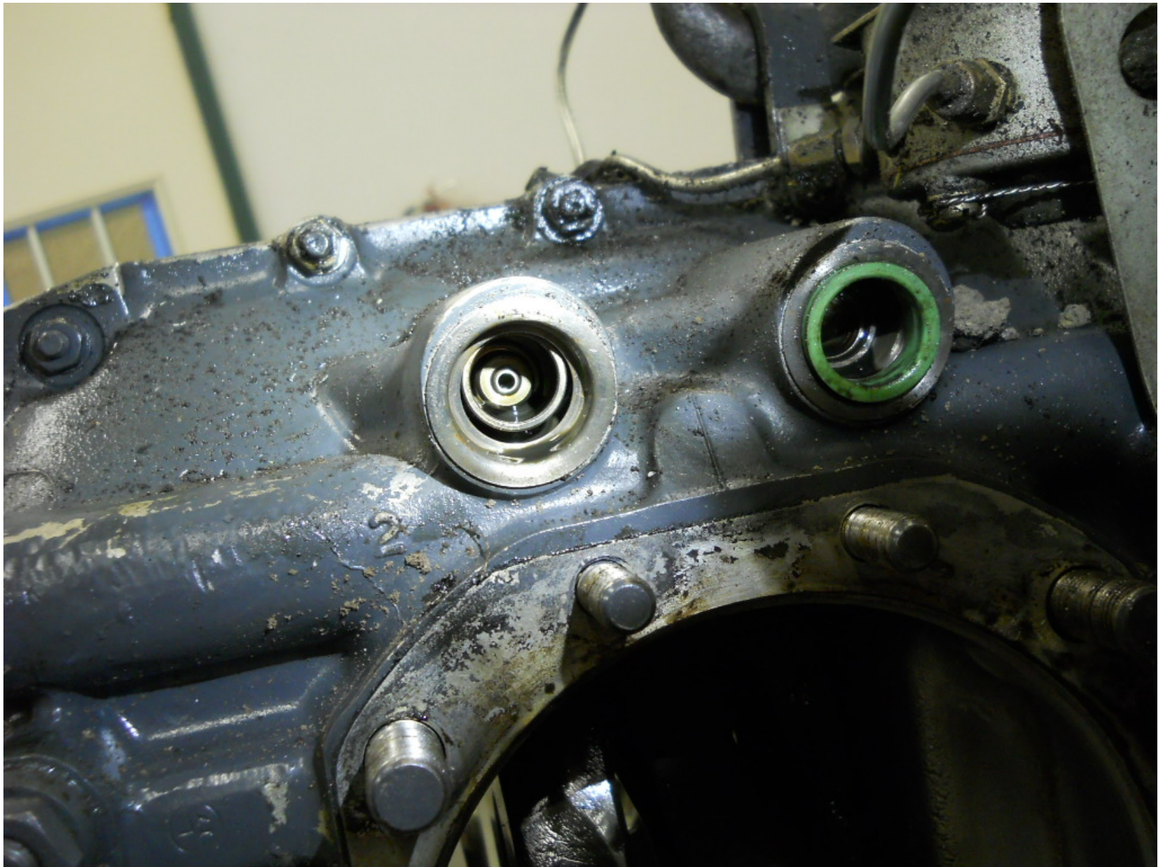
Photo 3 - #2 Cylinder with View of Improperly Installed Tappet (NTSB)
