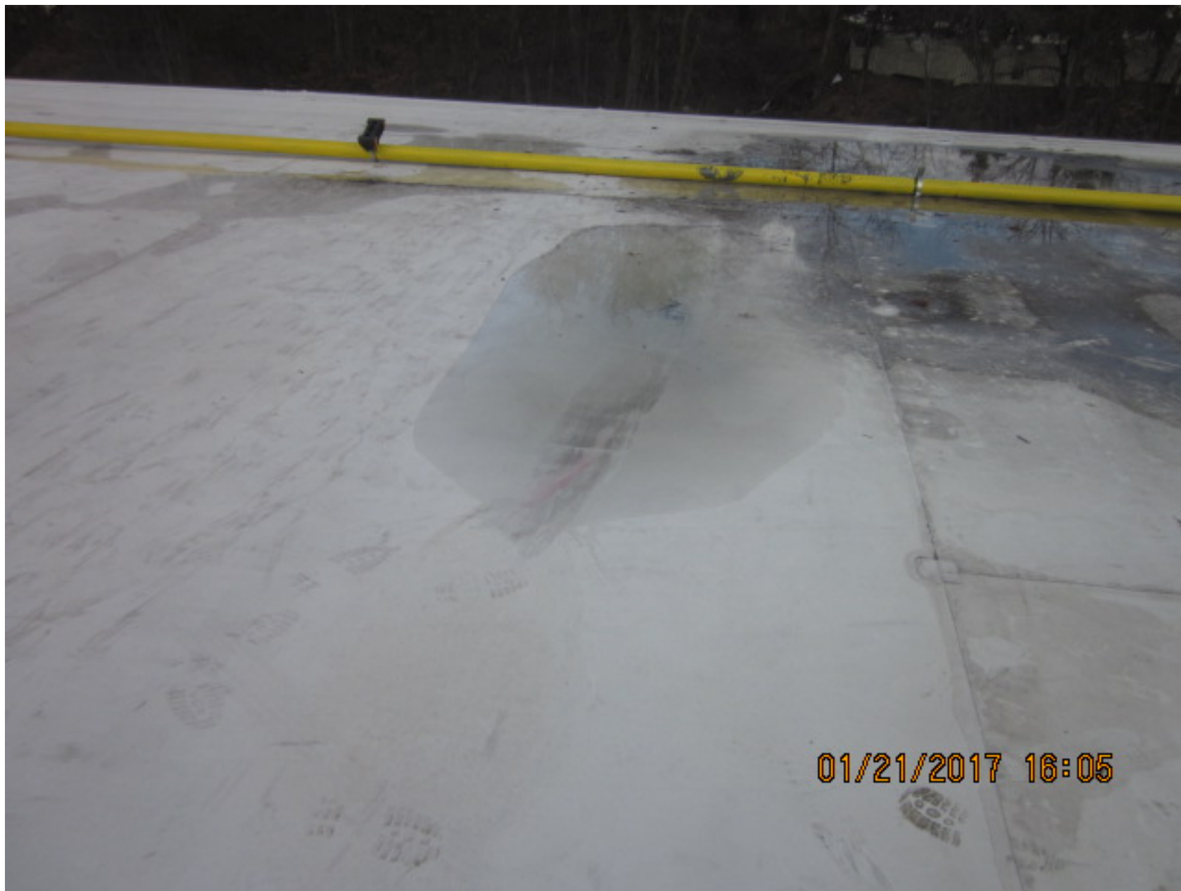
Photo 1 – Point of Contact on Roof of Building – Courtesy of FAA
