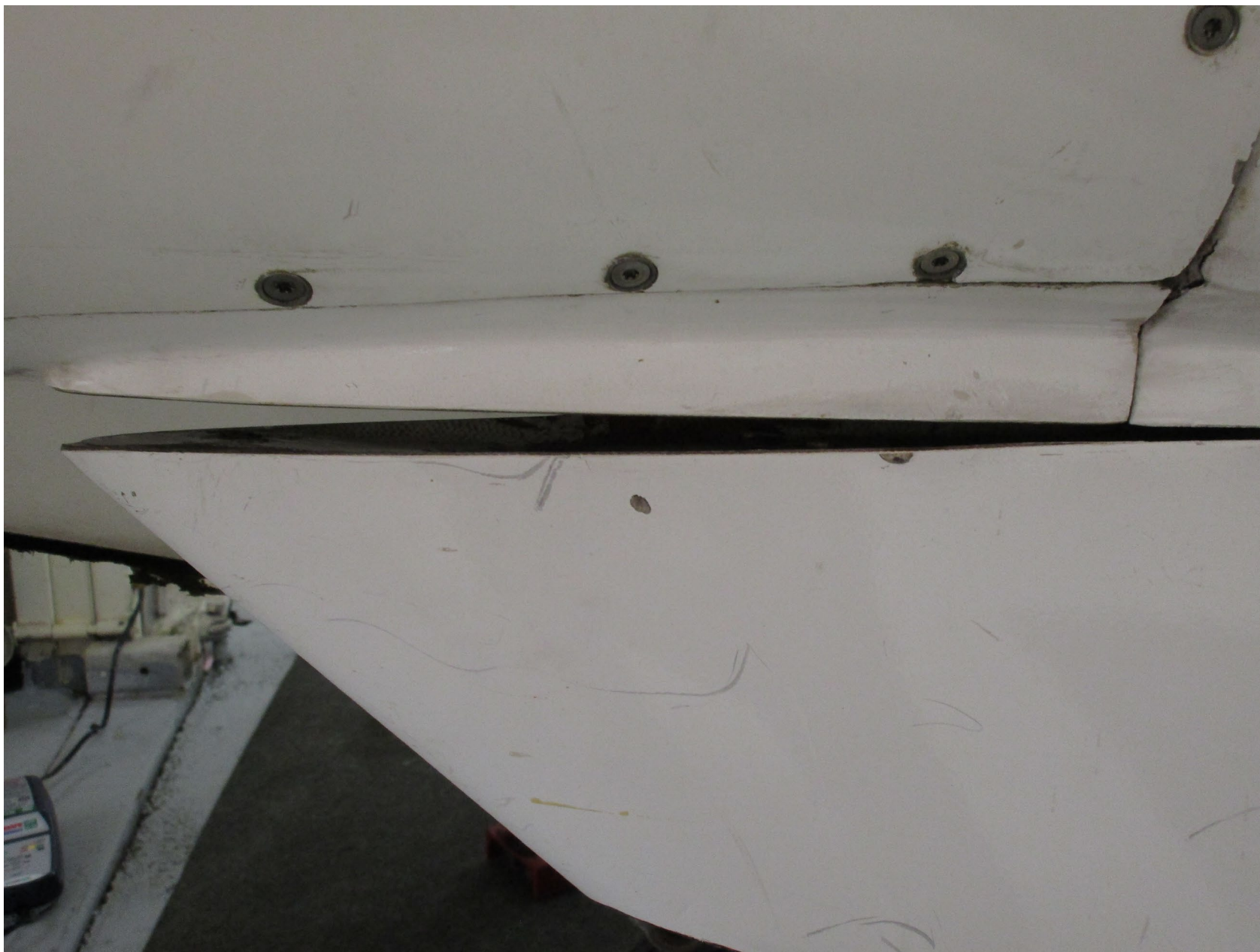
Photo 9 – Gap in Rudder / Fuselage Juncture – Courtesy of FAA
