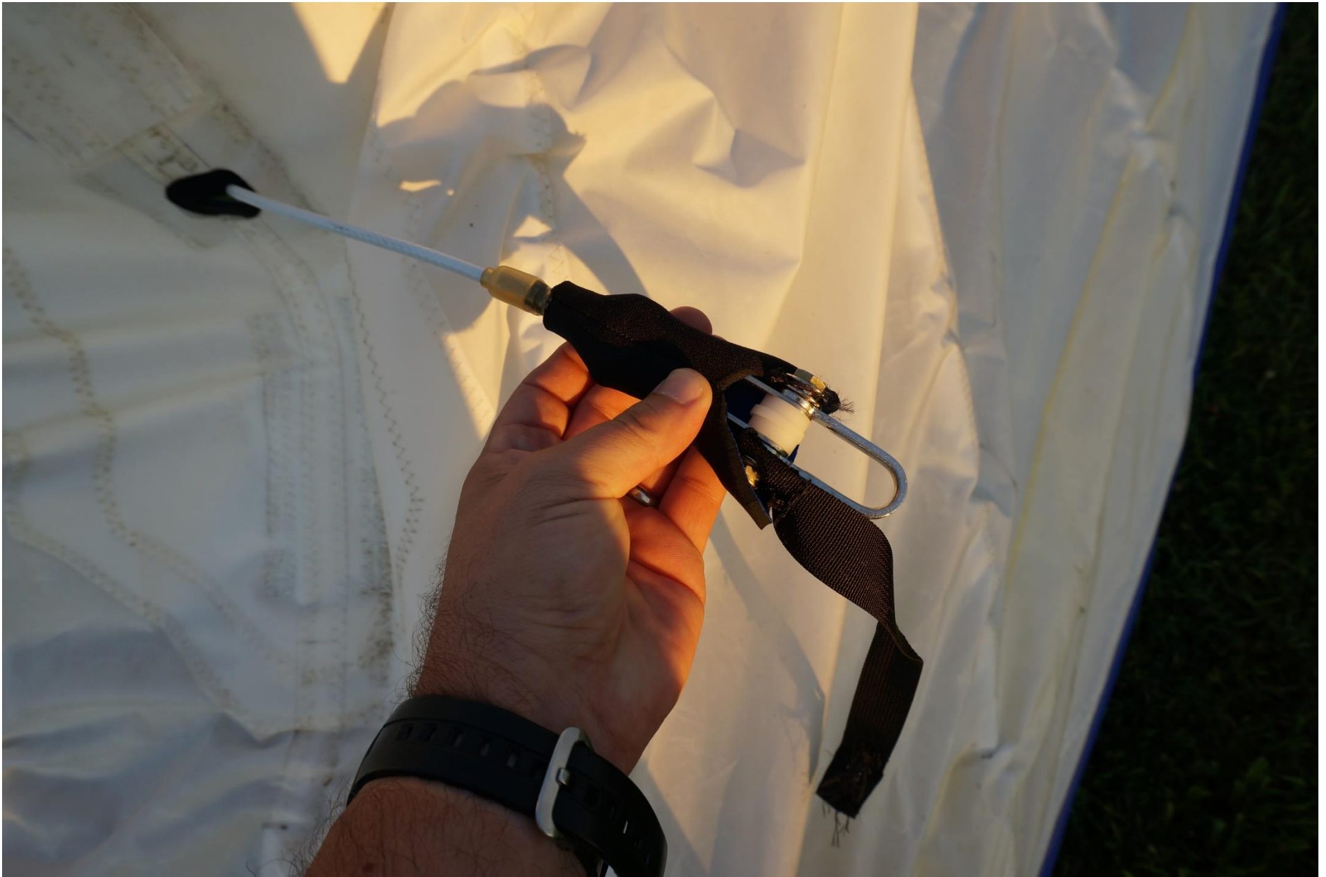
Cross Bar Restraint Cable – Aft End – As Found
