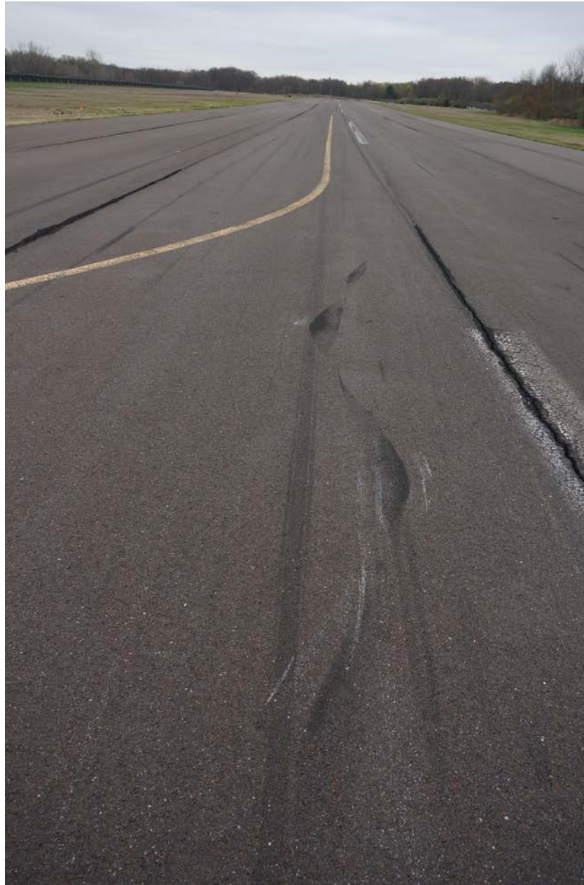
Photo 16 – First Set of Nose Wheel Tire Marks and Wheel Pant Paint Transfers
