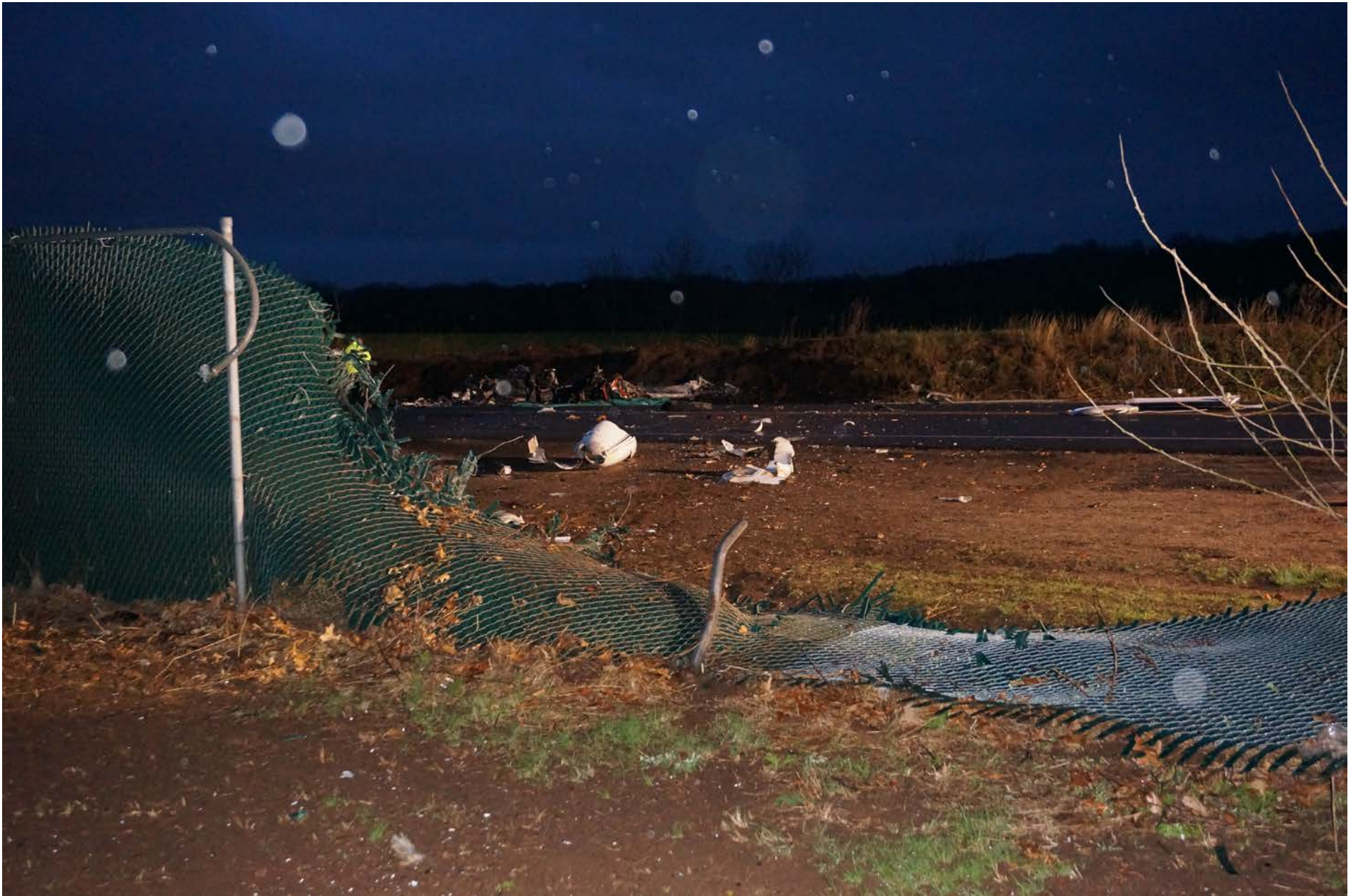
Photo 1 –Breach in Airport Security Fence
