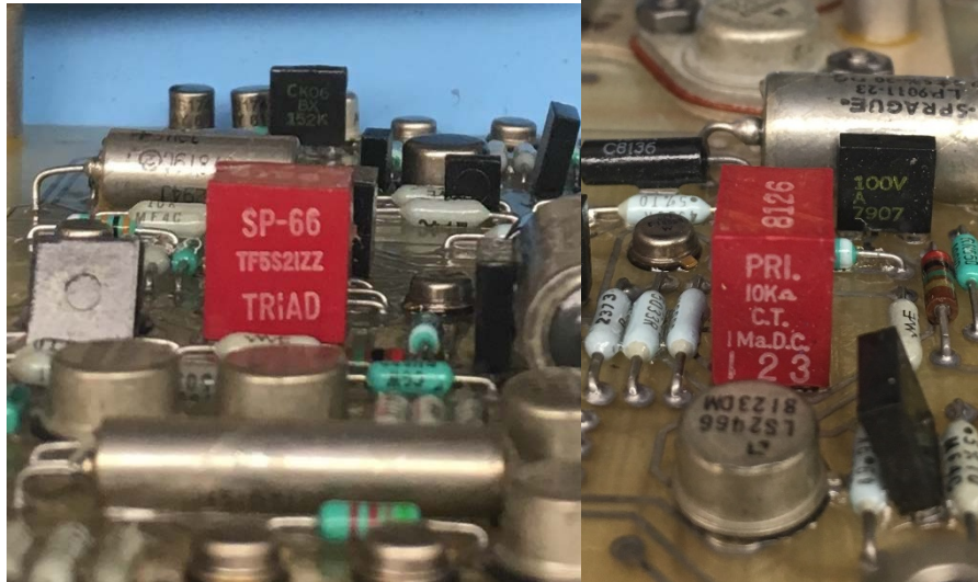
Figures 13a and 13b – Views of the "Red Transformer" prior to removal from an ancillary Pitch CCA by Duncan Aviation.
