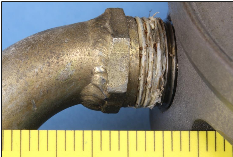
Figure 2. Close view of the outlet tube partially unscrewed from the housing. Teflon thread tape was present on the threads.
