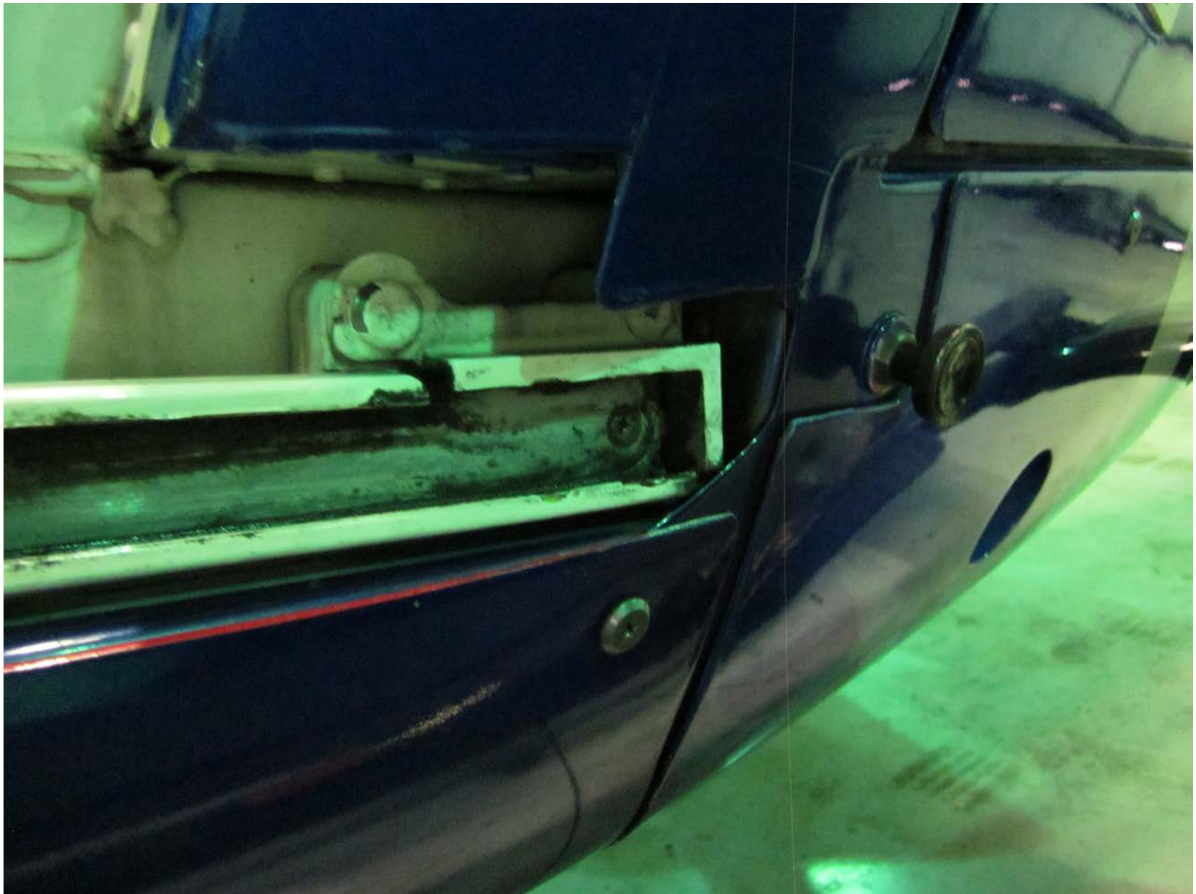
Photo 3 – View of lower door track
